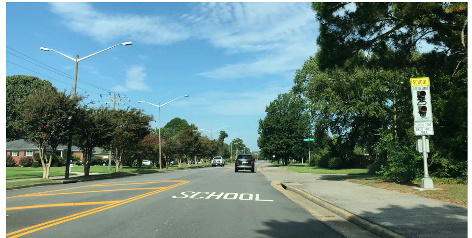
Sidepaths, like this one on Inlynnview Road, provide space for walking and bicycling but do not have a buffer.
