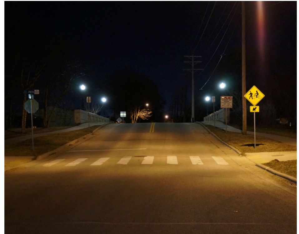
Figure 72: A well-lit mid-block pedestrian and bicyclist crossing and sidewalk with pedestrian-scale lighting
