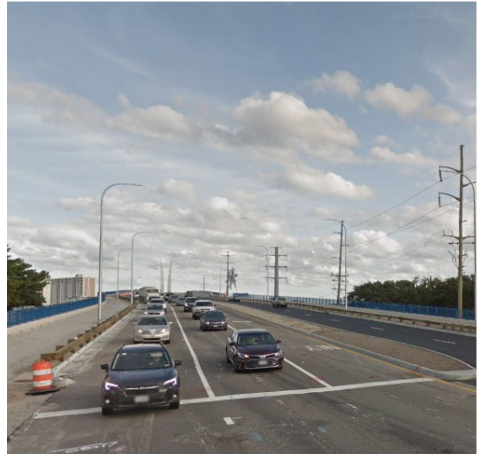
Figure 71: Lesner Bridge in Virginia Beach accommodates pedestrians and bicyclists with separated facilities
