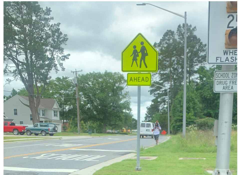
Gaps in sidewalk connectivity on Seaboard Road force pedestrians into roadway.
