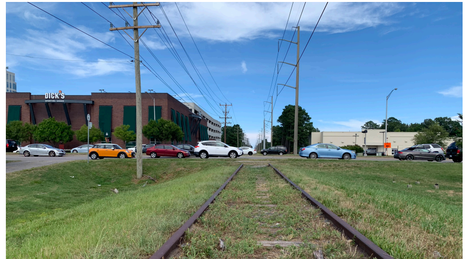
Future Virginia Beach Trail within city-owned transportation corridor (former NSSR Corridor).
