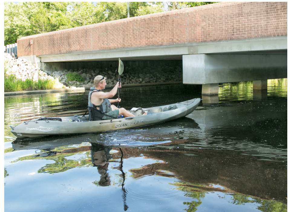
Bridges can accommodate blueway travel if designed with clear zones for kayaks and canoes.
