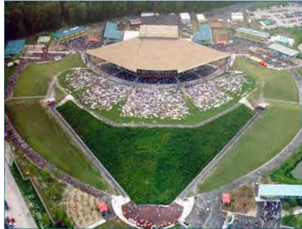
Amphitheater in North Princess Anne Commons Area
