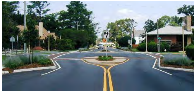
Street Calming in the Old Beach Neighborhood
