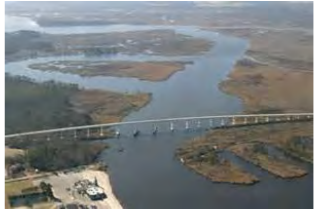
Pungo Ferry Bridge over North Landing River (AIWW)
