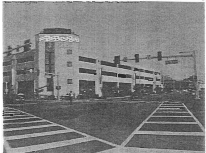
Figure 18: Existing parking garage at the beach front resort area.
