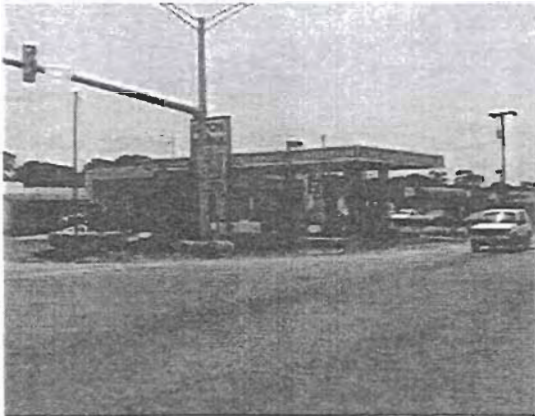
Figure 14: Poor driveway location on Shore Drive adjacent to existing intersection.
